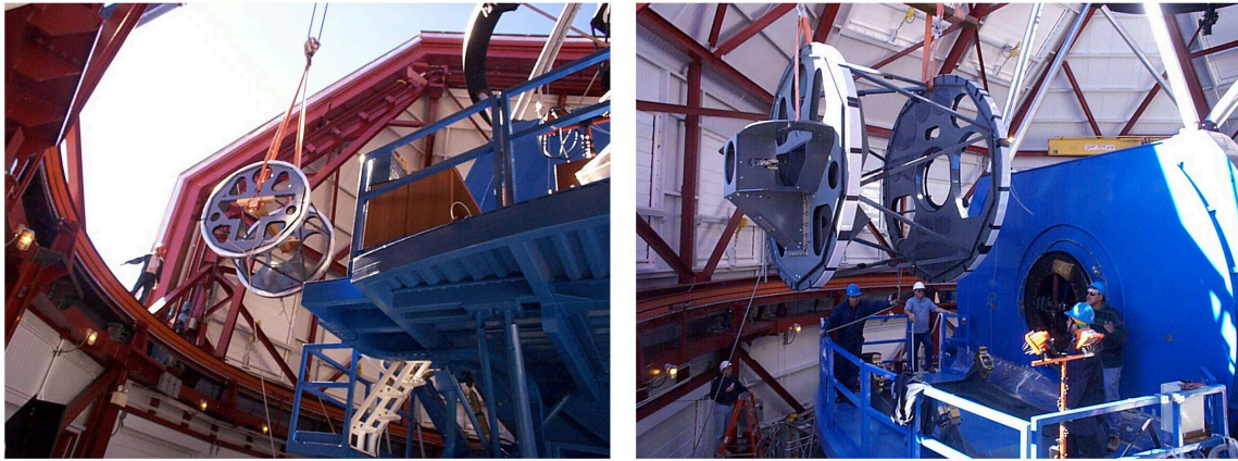
Fig. 37. (left) In August 2003, IMACS is raised from a palette outside the Magellan enclosure by the dome crane and lifted through the dome slit. (right) IMACS is positioned on the west Nasmyth platform.
